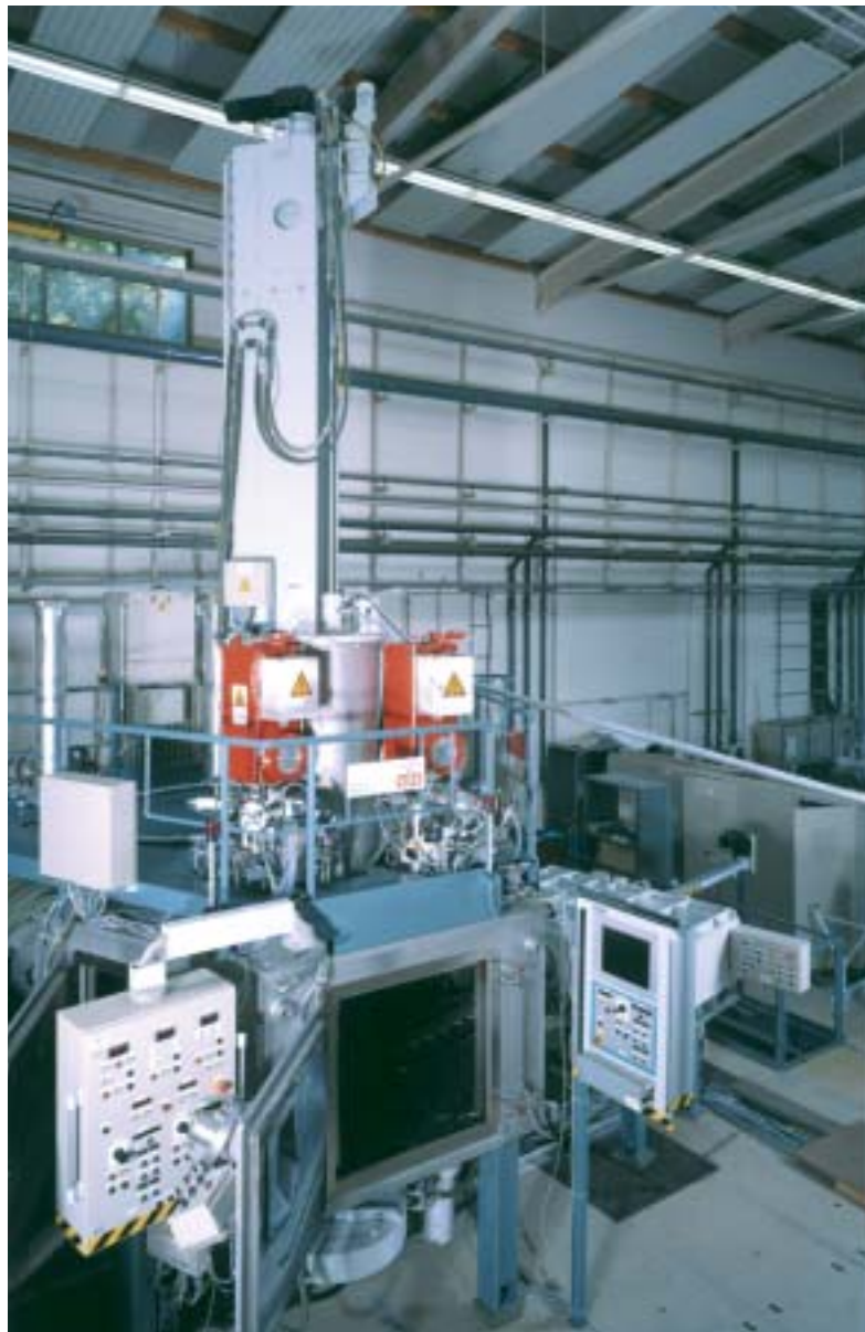
Front access door of EB Melting Furnace.
